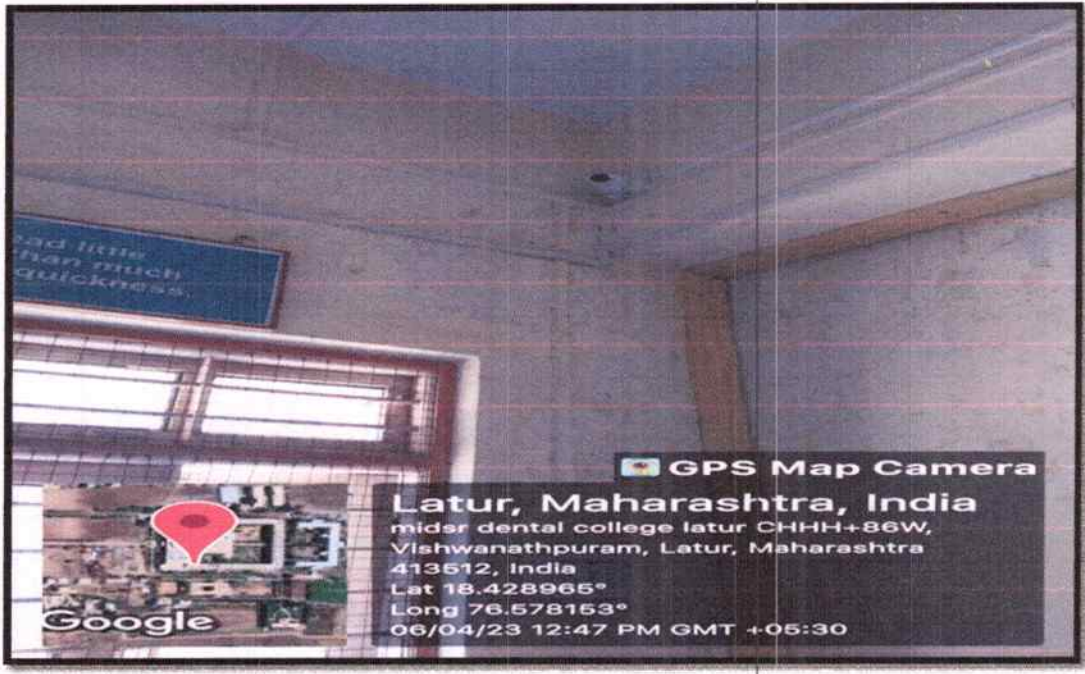
CCTV Surveillance inside the campus
